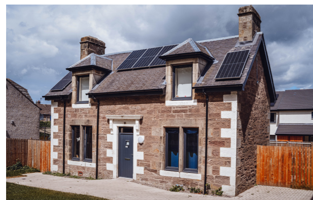
Crieff Road, Perth - 1 unit (existing house) - completed July 2022 (phased completion, 6 units completed in 2021-22)
