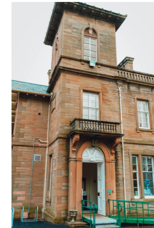
Bowerswell House, Perth - 3 additional units- completed March 2023
